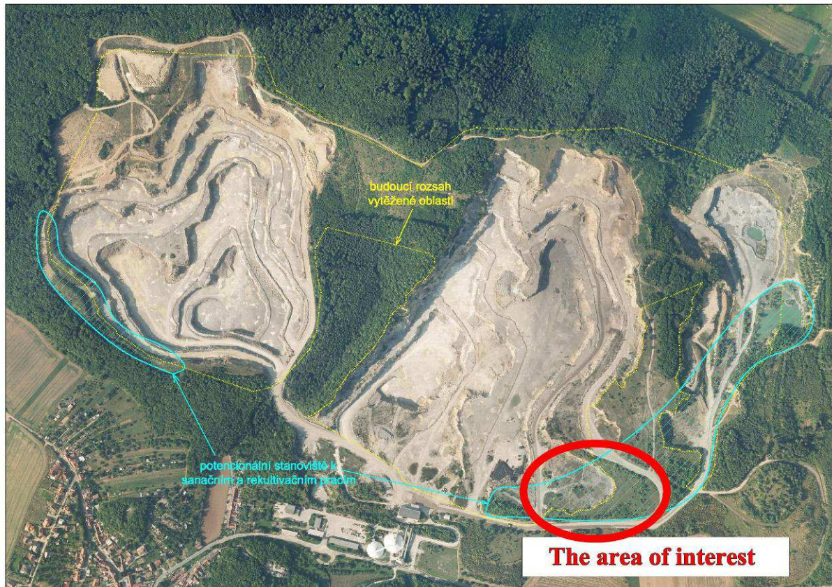
Appendix 1: The area of interest, the locality “Mezi lomy” in the right side and the formerly mined horseshoe-shaped area suitable for restoration in the left side of the red ellipse.
