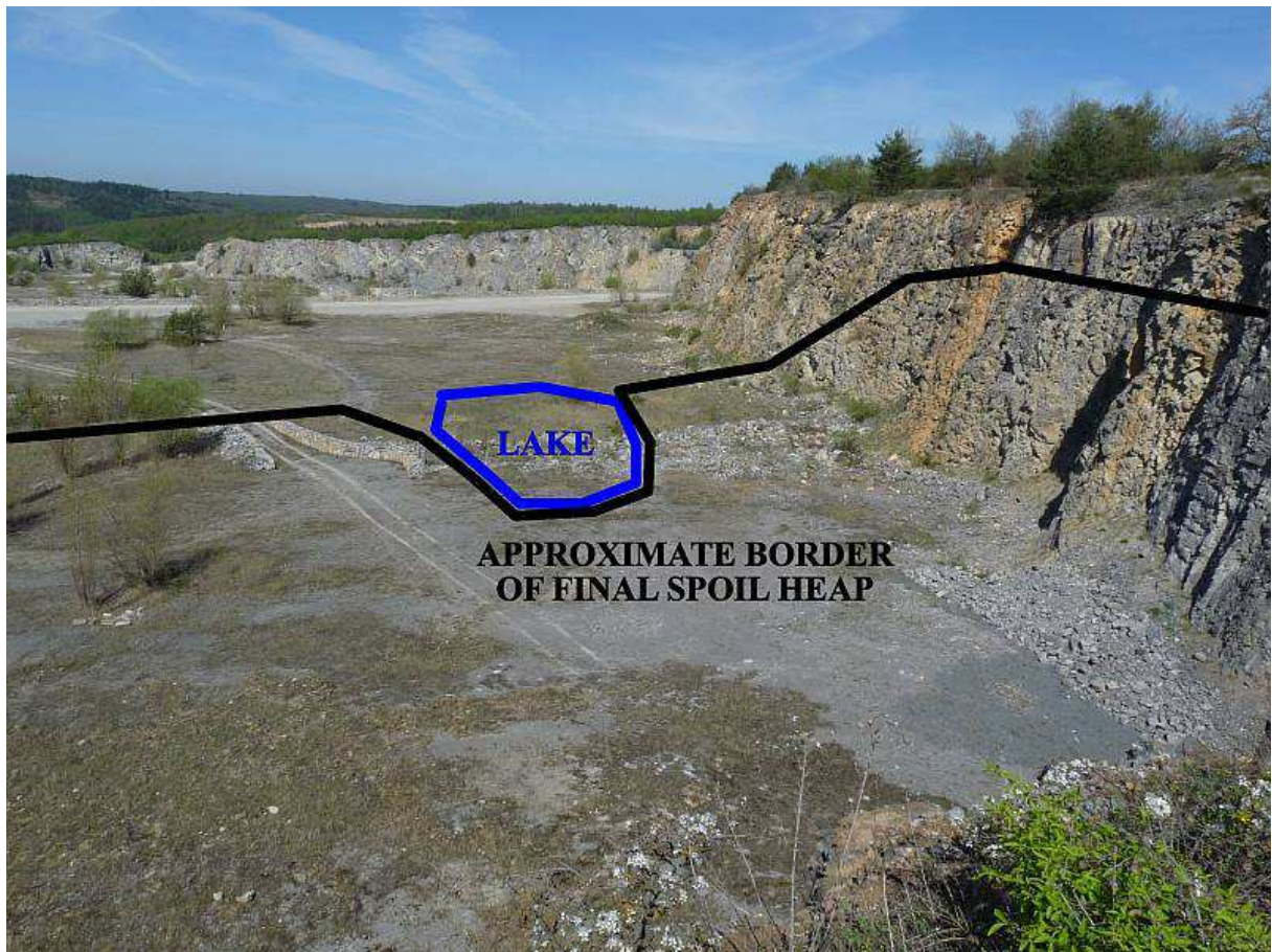
Appendix 28: The outline of final spoil heap approximate border, the upper level of heap should lay 2-3 m below the upper rock faces edge, 27.4.2012.
